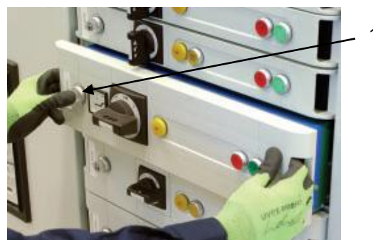
Fig. 5-5 Withdrawable unit with mechanical test position button
