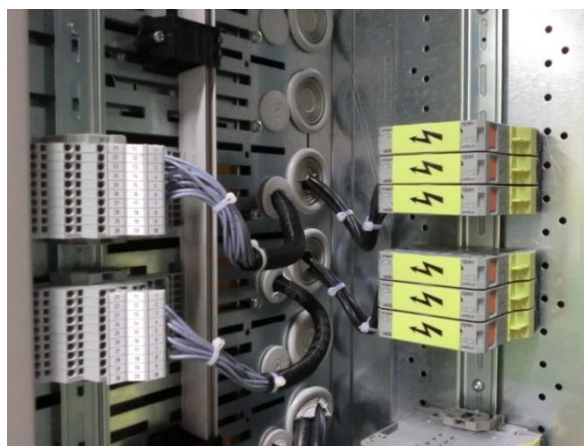
Fig. 3-17 Cable connection for withdrawable units
