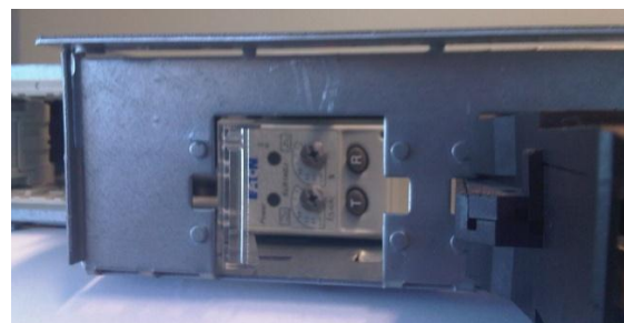
Fig. 3-12 Earth Fault Relay settings adjustment (2)
